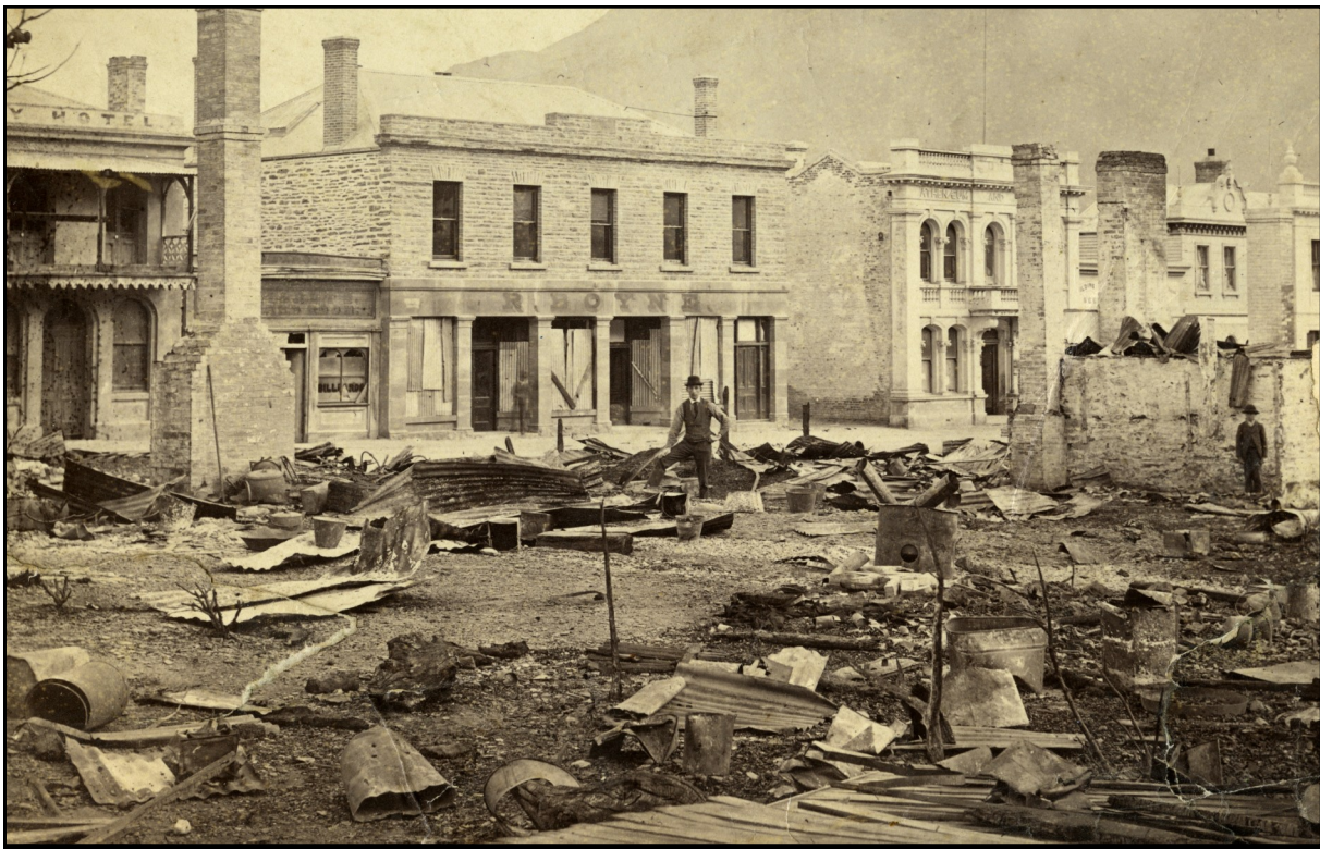
Ballarat Street after the fire
